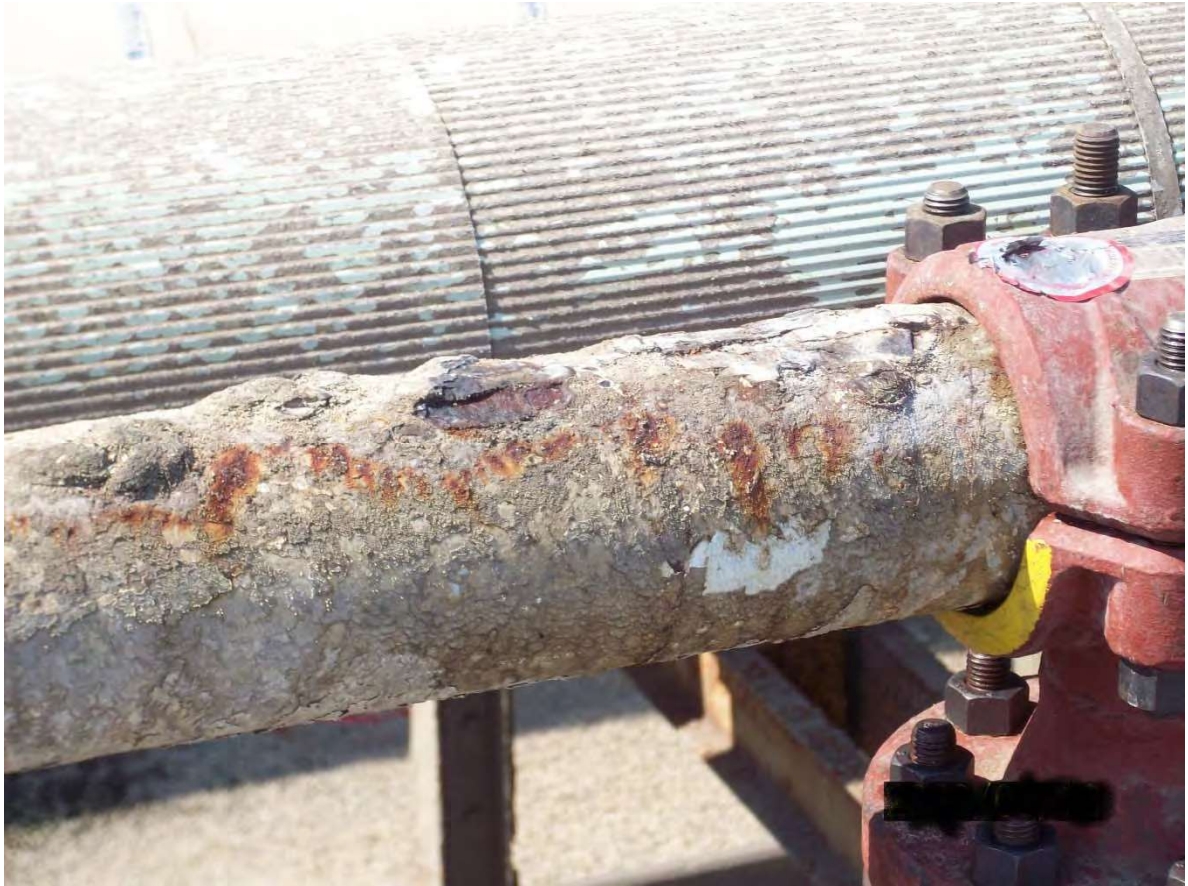
Figure 3-8-1—Atmospheric corrosion of an LPG line in close proximity to a cooling tower.
