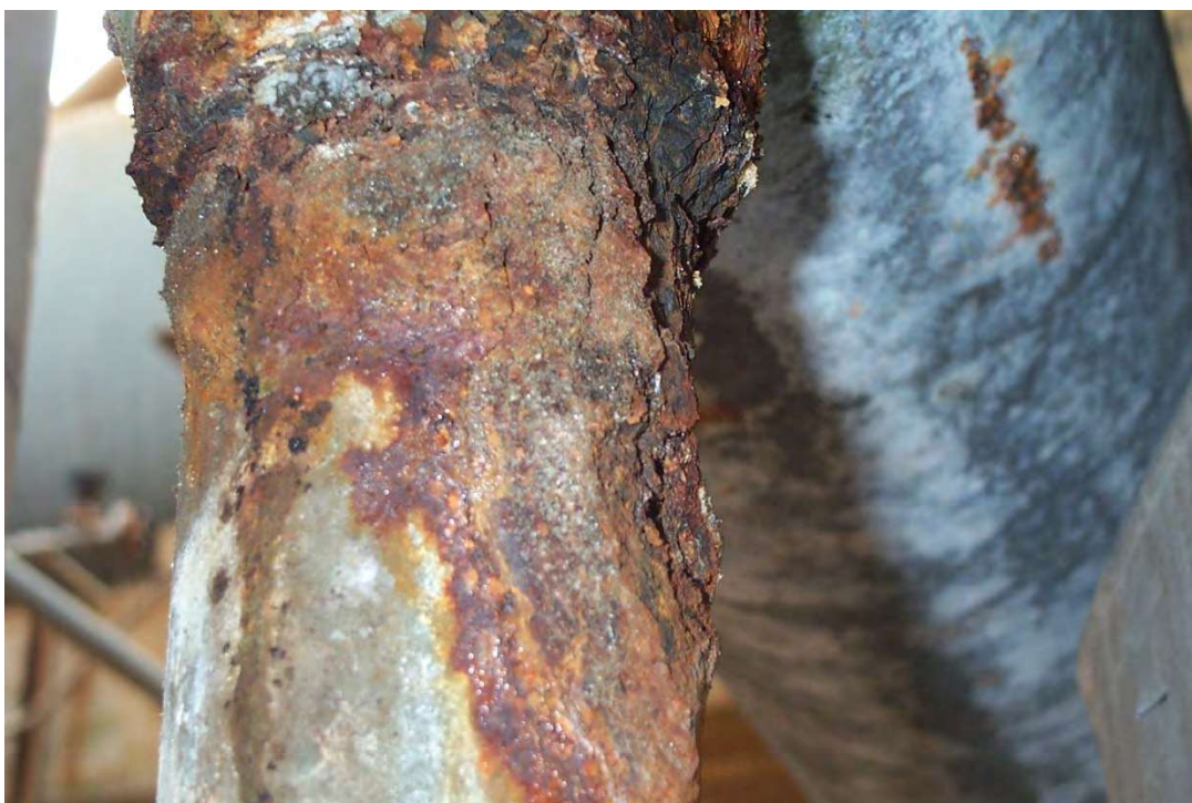
Figure 3-22-2—Close-up of the tee in Figure 3-21-1 after insulation removal.
