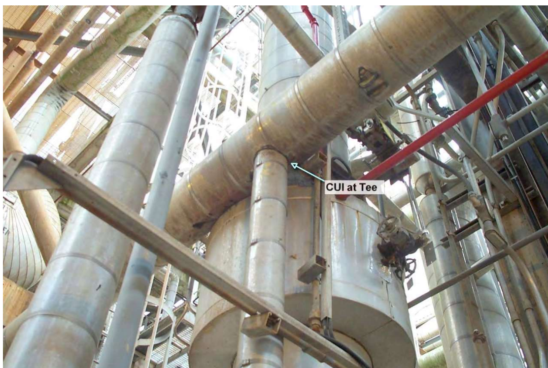
Figure 3-22-1—Piping tee in a 1000 psig ethylene line before insulation removal.
