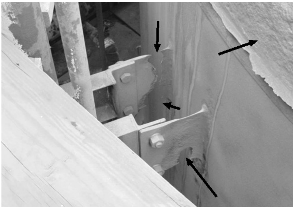
Figure 3-22-7—CUI at attachment supports and on the vessel head.
