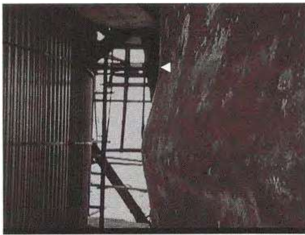
Figure 3-64-3—Bulging in a skirt of a coke drum due to thermal cycling from coker operation.
